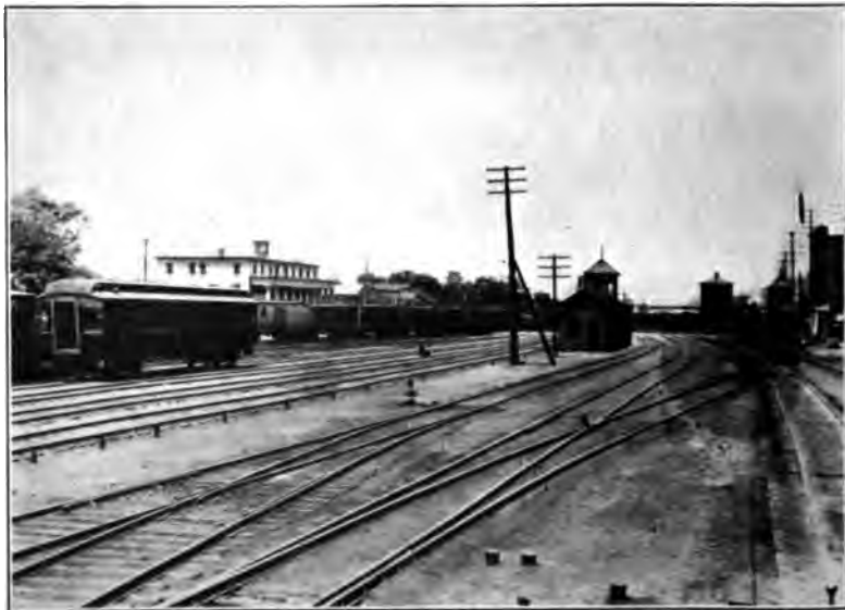
THE YARDMASTER'S OFFICE — IN AN ABANDONED SWITCH-TOWER
